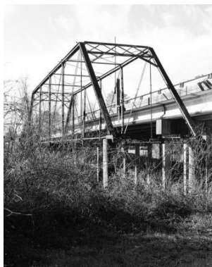
San Jacinto River 1910 Truss Bridge
